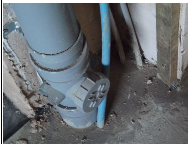
P18) Foam around floor edge trimmed back and then parged over to seal before final test
