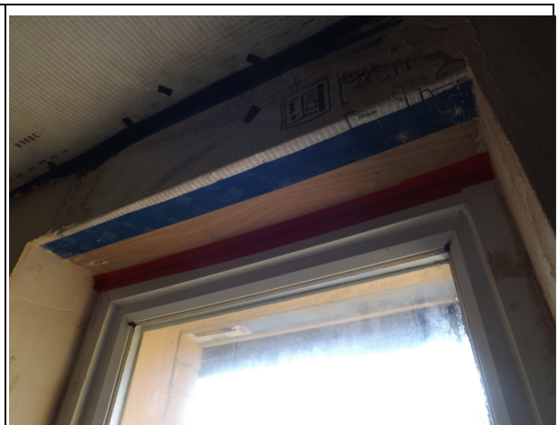
P12) Red tape sealing crack across top of existing window
