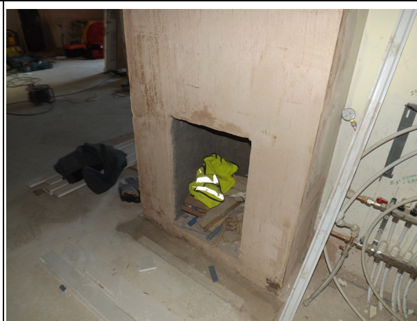
P14) Fireplace completely parged before final test
