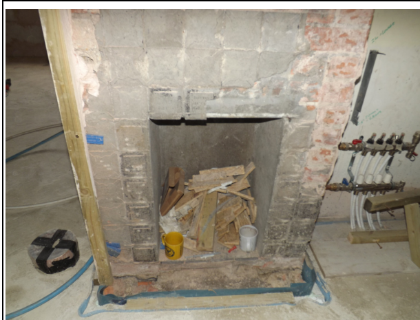
P13) Leakage in various gaps in brickwork at locations around existing fireplace
