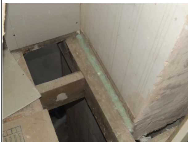
P15) Expanding foam used to seal void behind intermediate floor joist near existing chimney
