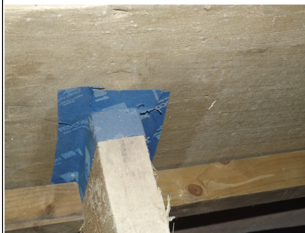
P16) Tape seal around end of floor joist into wall
