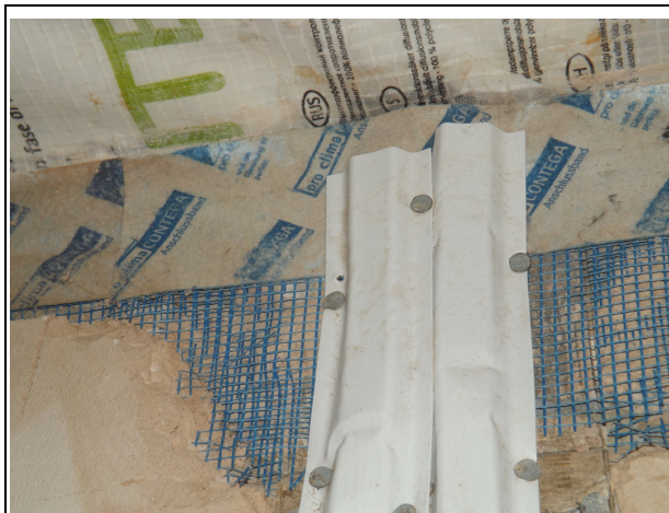
P11) Leakage behind conduit, removed and wall parged before final test
