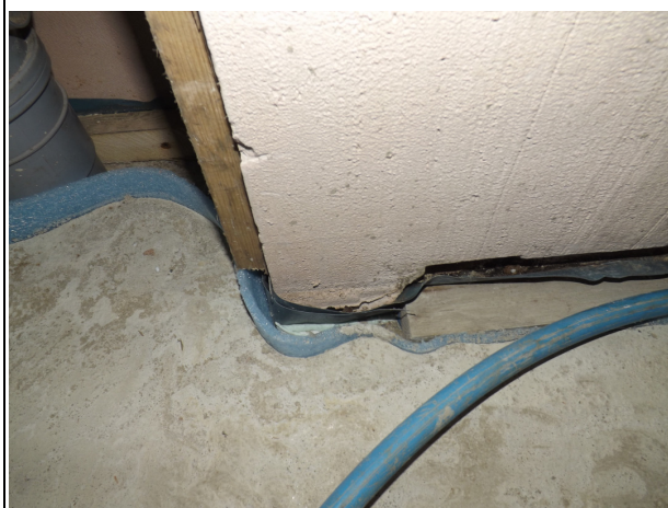
P17) Leakage found at edge of floor behind existing chimney
